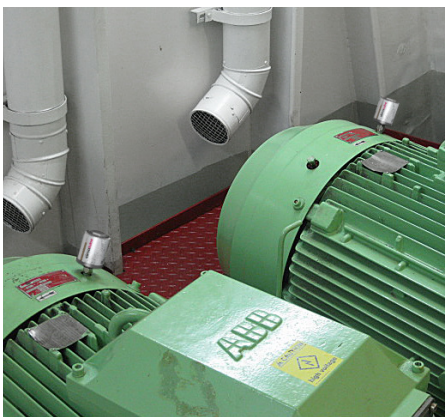
The ABB electric motors are fitted with 60 ml simalube lubricators.
