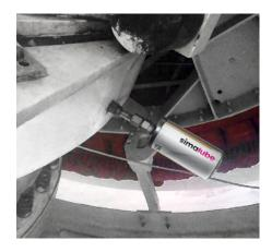
In this wind turbine, the simalube lubricator is set with a dispensing time of six months.
