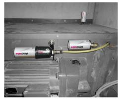
The lubricant is fed to the lubrication point via a long line. A mounting bracket with two magnets fixes the simulube IMPULSE connect to the machine.
